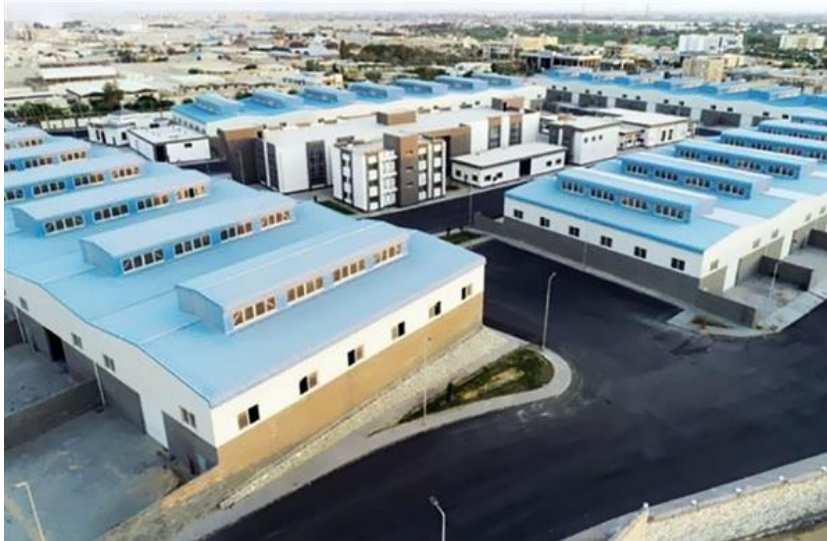
28-SITE WORK FOR EXECUTION SUPERVISION
