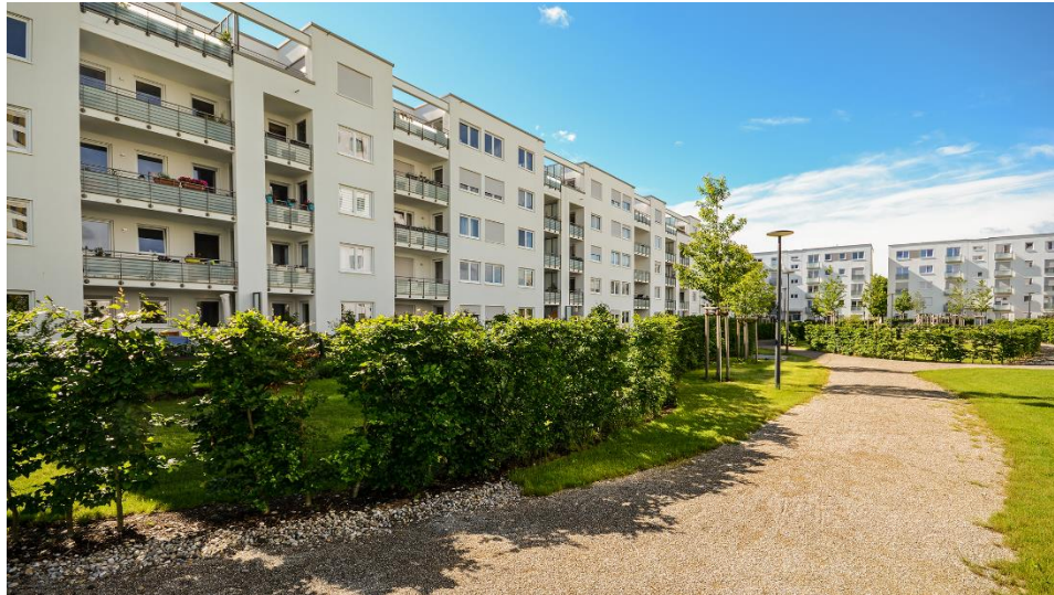
29-EXTERIOR SITE SHOT
